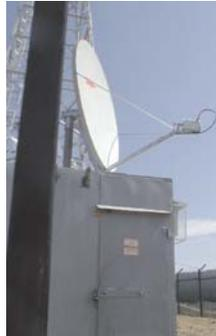
One area of the new standard relates to the environmental and electrical conditions found outdoors. The standard includes a section covering elevated ambient temperatures, increased exposure to transient overvoltages and the possible rise of earth potential.
